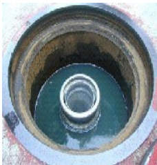
Liquid in spill bucket
