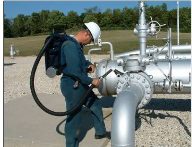
Leak Measurement Using High Volume Sampler
