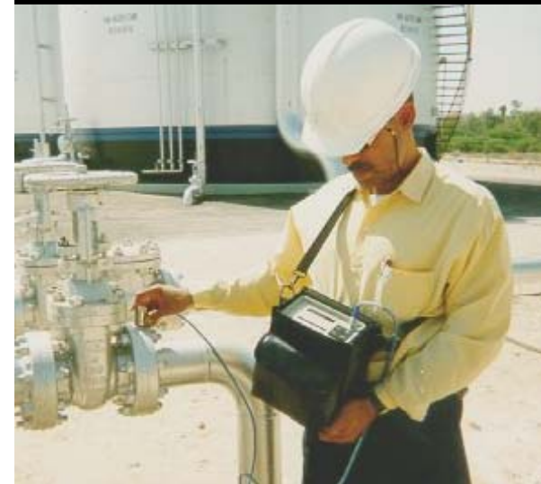
Acoustic Leak Detection
