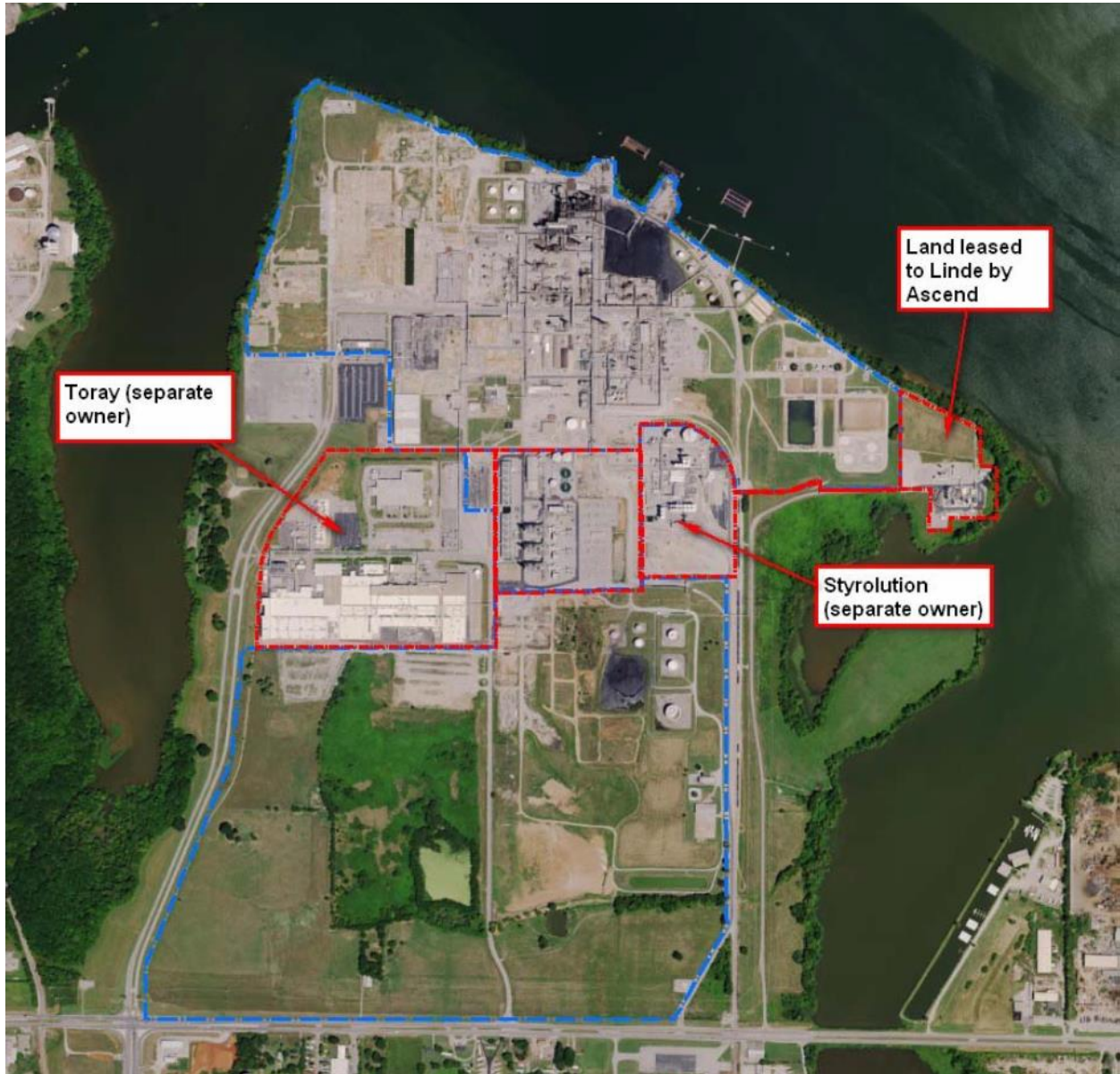
Figure 39. Areas Fenced by Other Industry. Source: “Air Dispersion Modeling for Evaluating Compliance with the 1-Hour SO 2 National Ambient Air Quality Standard at the Ascend Performance Materials Facility in Decatur, Alabama” prepared for Alabama, December 2016
