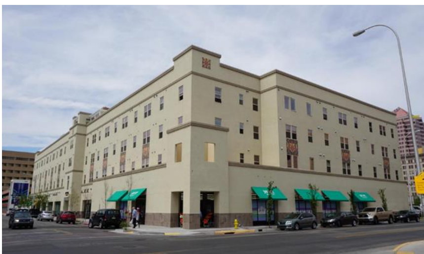
Completed 12,000-square-foot grocery store sits on a former brownfield site in Albuquerque, New Mexico. (EPA photo)
