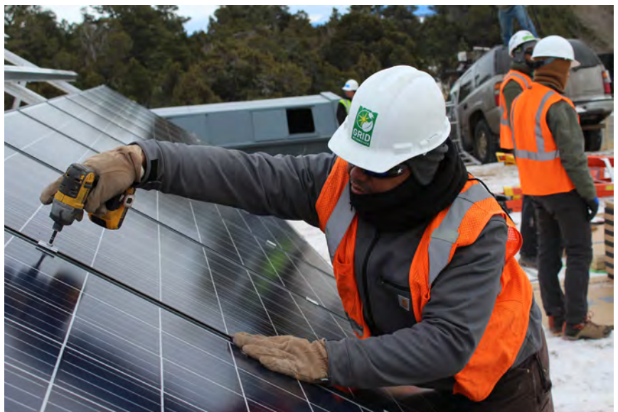
Installation of the San Miguel community solar array in Norwood, Colorado.
