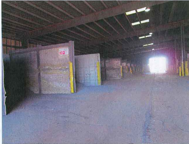
Indoor Bulk Material Storage Bay
