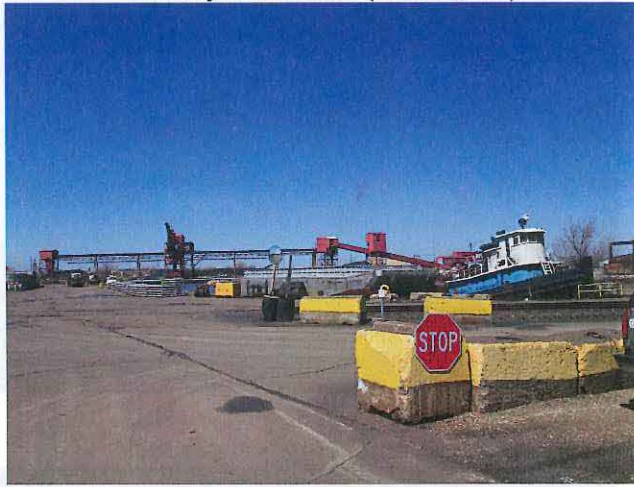
Facility Overview (West view)
