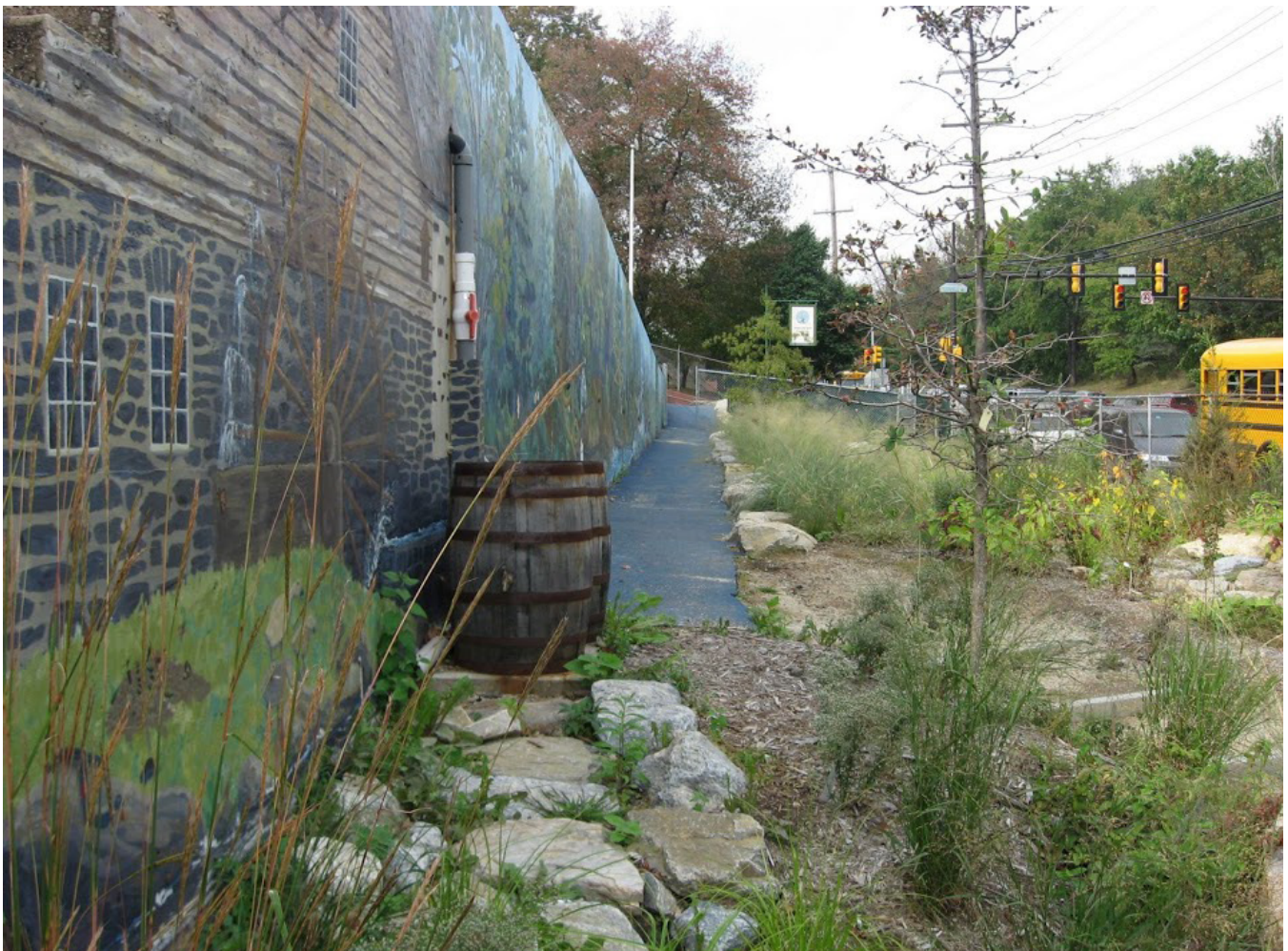
Green stormwater infrastructure includes a wide range of approaches, including rain barrels, which catch rain water for plants instead of running off into storm drains and streams.
