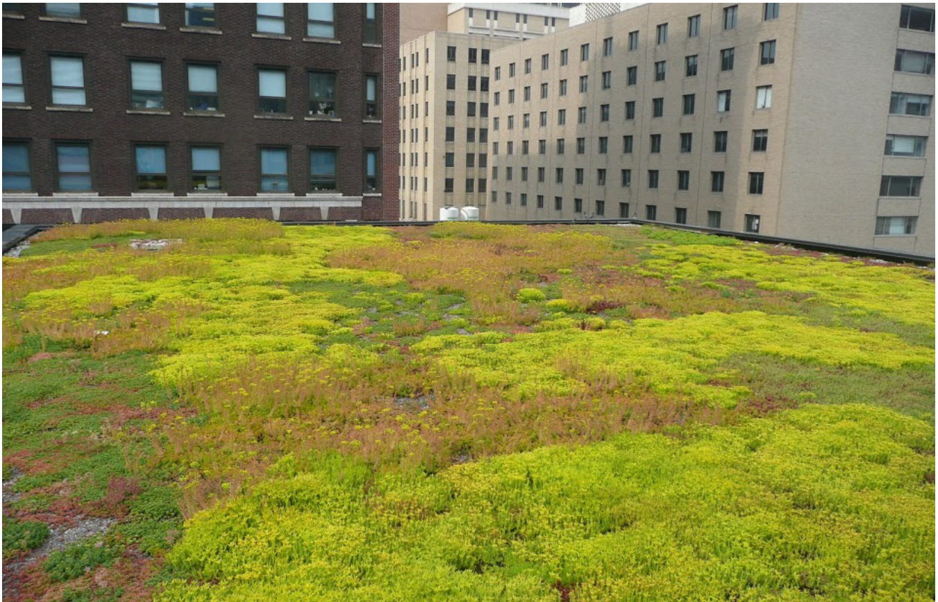
Green roofs can reduce and slow stormwater runoff in the urban environment; they also filter pollutants from rainfall.
