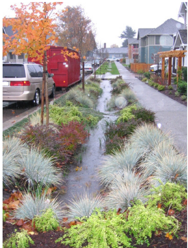
Techniques such as rain gardens, like this one in the High Point neighborhood in Seattle, WA, retain stormwater runoff, which can help reduce peak flooding.
