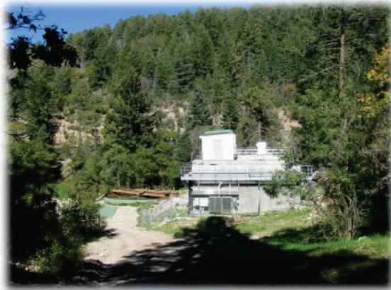
Figure A.4-1. Wastewater treatment plant
