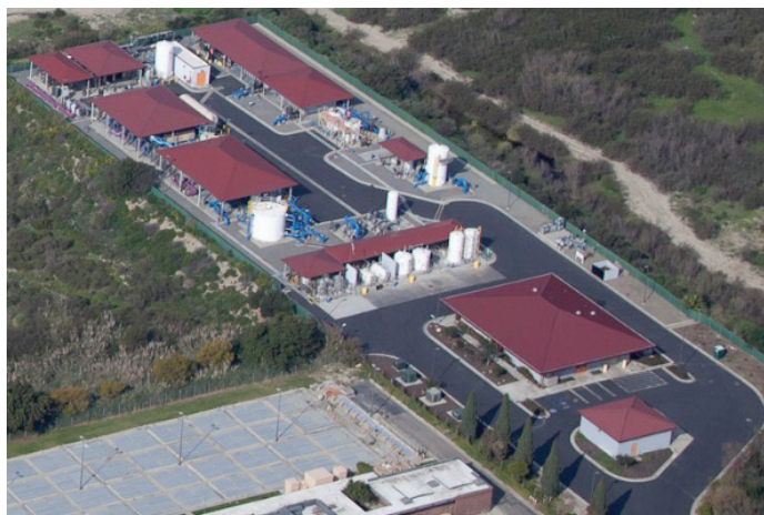
Figure A.1-3. Leo J. Vander Lans Advanced Water Treatment Facility (WRD, 2015)
