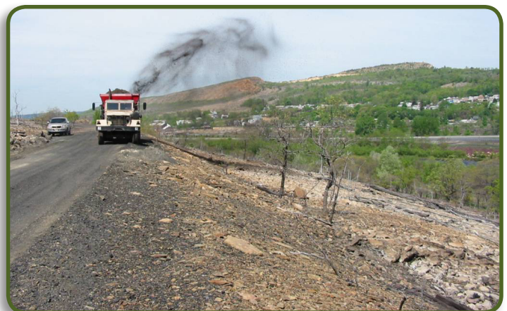
Soil amendments applied using a spreader truck
