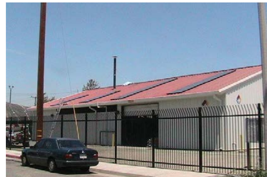
PV Green Remediation at Pemaco, CA Superfund Site
