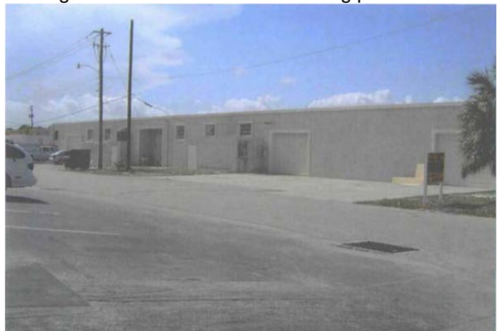
Treatment Plant #1, Hollingsworth Solderless (EPA, 2011a)
