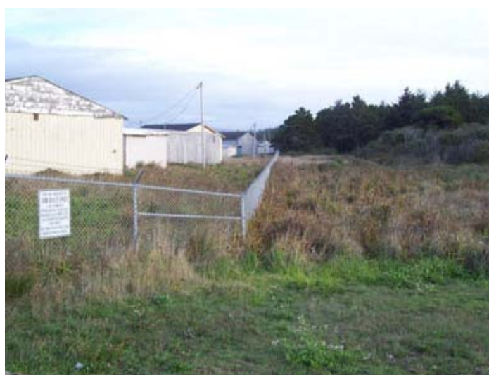
Del Norte Pesticide Storage Site (right) and Adjacent Airport (left) (EPA, 2010b)
