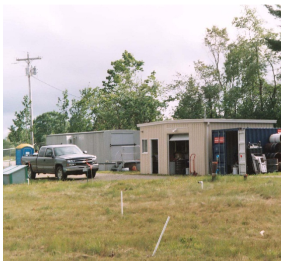
Treatment Building (EPA, 2011)
