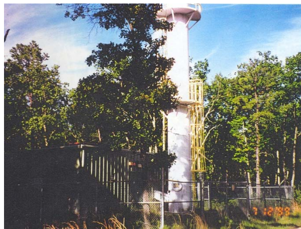
Treatment building and air stripper tower (Waste Technology, 1999)
