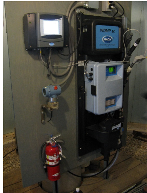
Figure 10-3. City of Dayton Water Department Monitoring Station Installation
