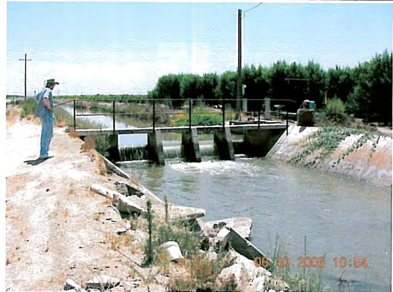
Drop structure in Banks Ditch.
