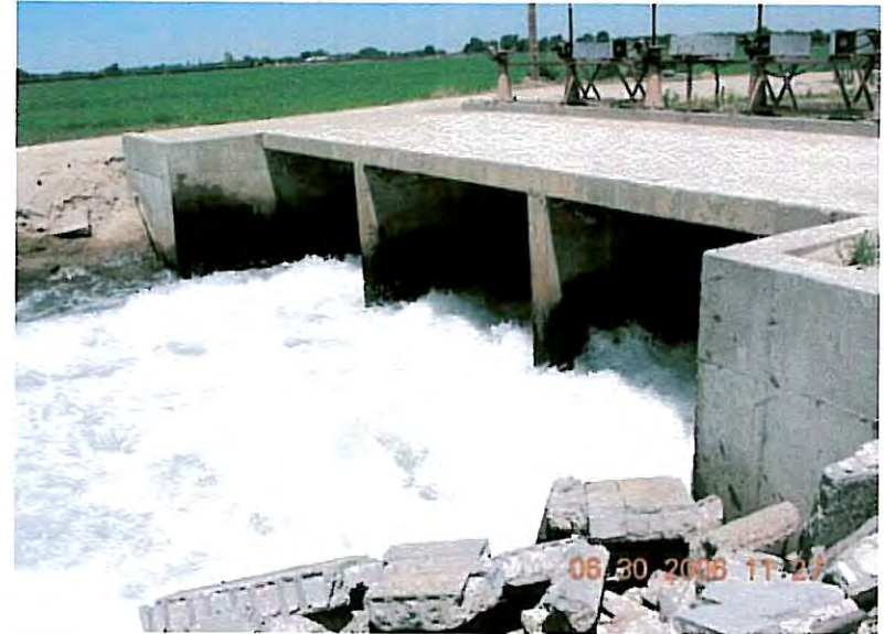
Drop structure in People's Ditch.
