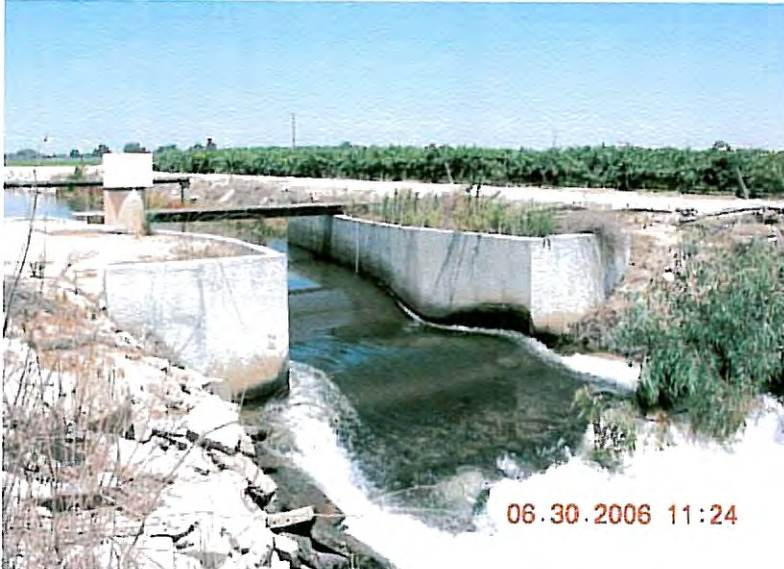
Flume on unnamed canal near People's Ditch.
