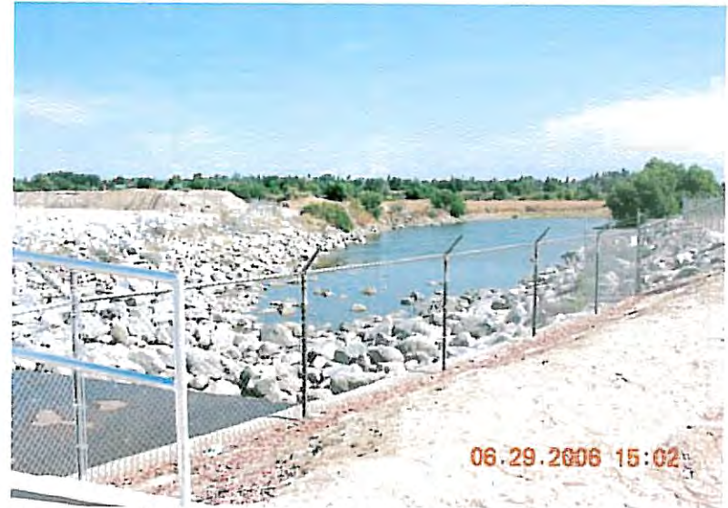
Channel connecting the Friant-Kern Canal to the Kern River.
