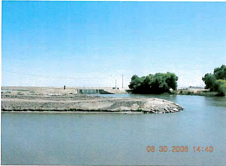
Kings River Canal south of structure on Kings River at Empire Weir No. 2.
