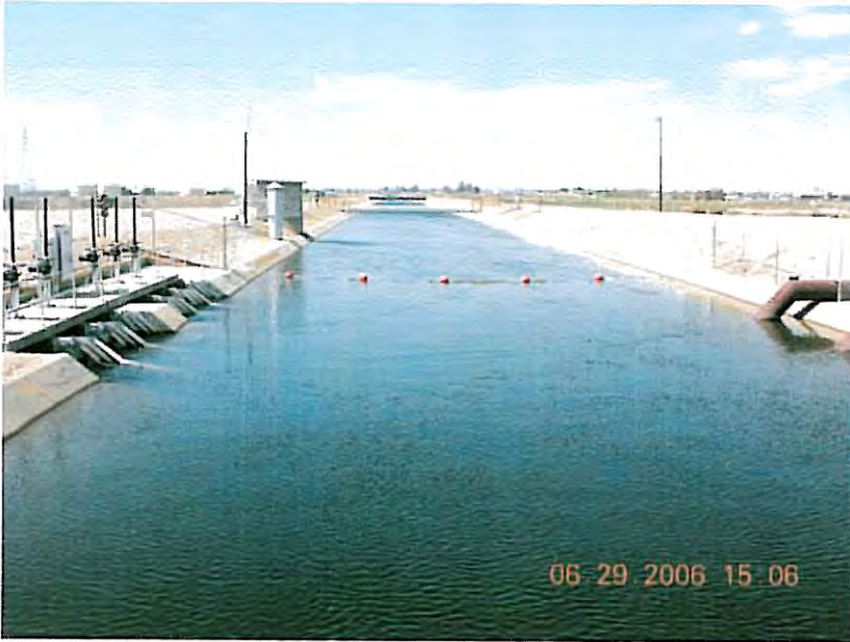
Friant-Kern Canal turn out into the Arvin-Edison Canal and siphon connection to the Cross Valley Canal.
