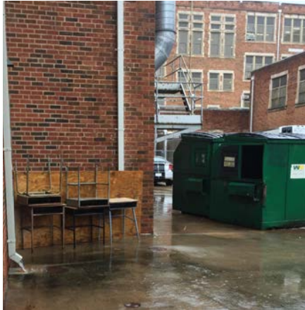
Figure 12. Rainwater from the school roof flows into the paved courtyard and contributes to flooding inside and outside the building.
