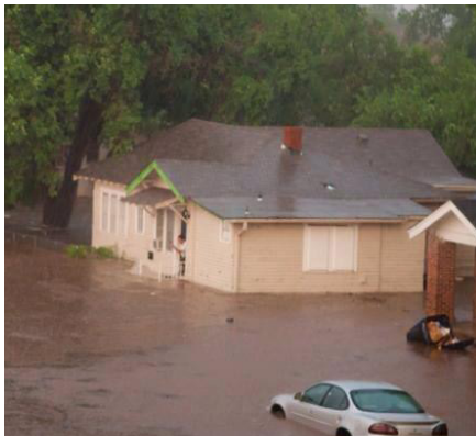
Figures 1 and 2. Images provided by Oklahoma City show flooding in project area neighborhoods.
