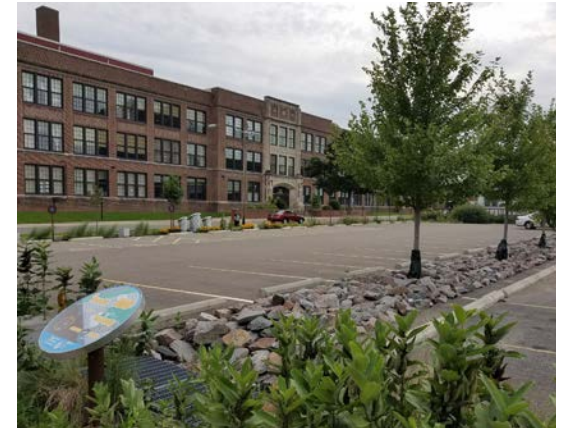
Figure 48. Pervious parking lot at Edison Green Campus.
