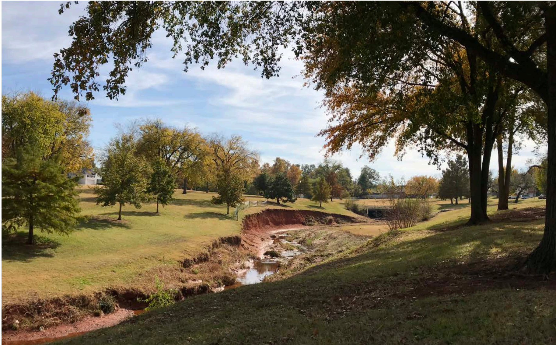
Figure 33. This image of Guy James Creek shows the severe erosion caused by high flow during rain events. The steep banks create safety hazards for park visitors.
