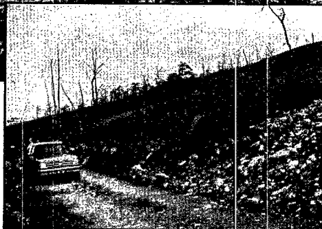
Above, truck spraying biosolids/fly ash mixture for revegetation at the Palmerton, Pennsylvania, hazardous waste site. Right, the same area after being reclaimed.
