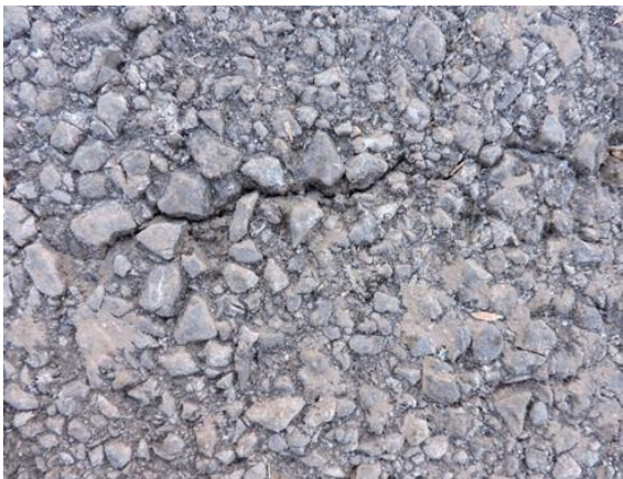
Parking Lot Asphalt
