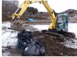
Topsoil stripping (mechanical digger)
