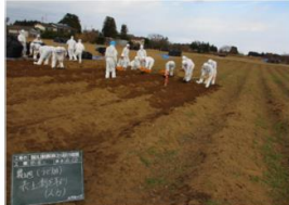
Manual topsoil stripping
