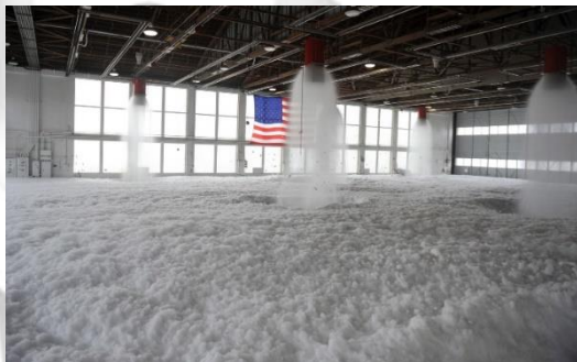
Aqueous Film-Forming Foam, or AFFF, fills Hangar 211 at Mountain Home Air Force Base, Idaho, Dec. 21, 2012. Photo: U.S. Air Force
