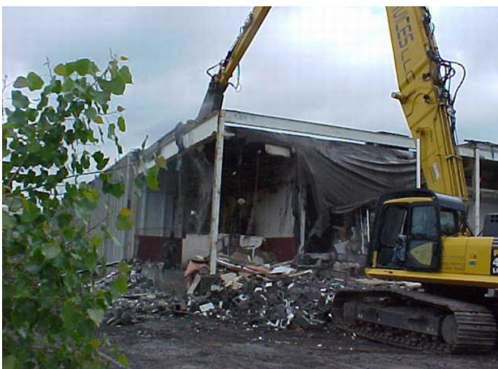
Removal actions included demolishing structurally damaged and contaminated buildings.
