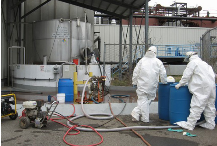
Cleanup of a sulfuric acid tank at the site (above) and the removal of chromic acid stored on the site (below).
