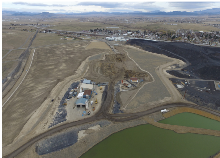
Aerial photograph of ASARCO property, East Helena, as of March 2016, is visible top right, near the ASARCO waste slag pile (black area on right).
