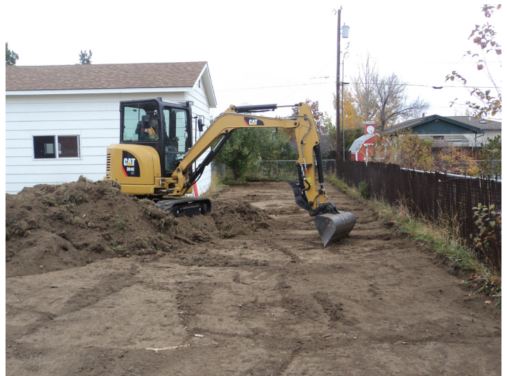
Residential cleanup in progress.
