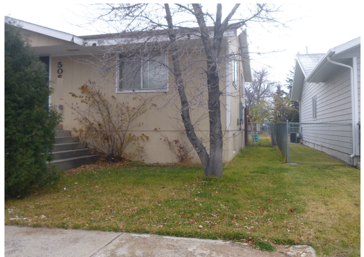
A remediated residential yard in OU2.
