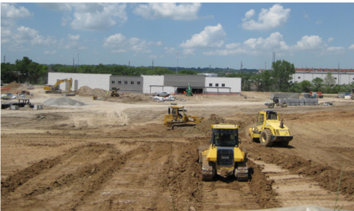
Construction underway on site for the Walmart Neighborhood Market.
