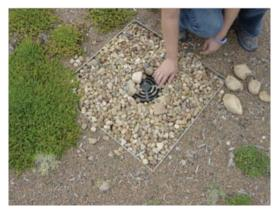
Image 31.1. Vegetation free zone around roof drain being cleaned out. Photo courtesy: Urban Drainage and Flood Control District.
