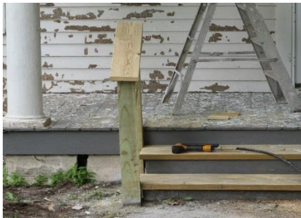
House with lead paint undergoing renovation. (EPA photo)
