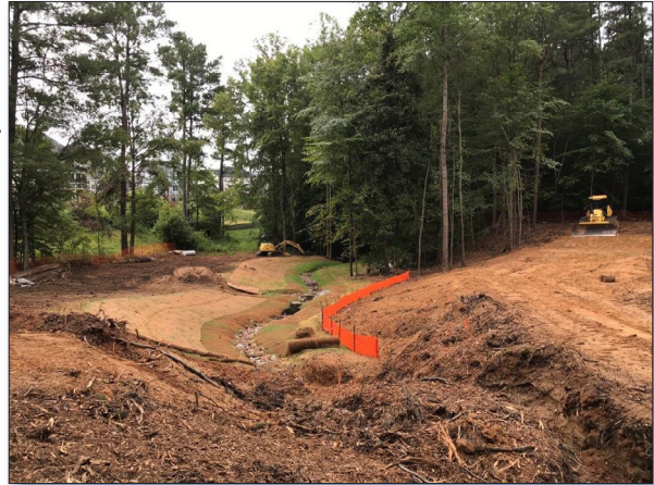
Figure 2. Partners completed an intermittent channel restoration project in the watershed.
