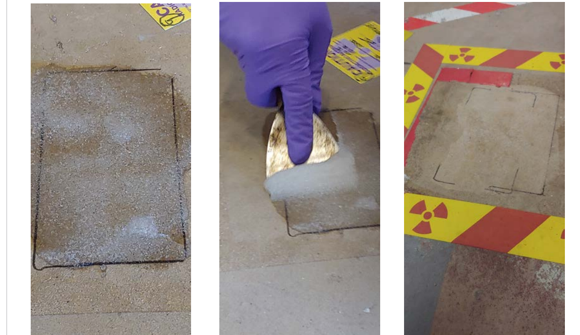
Argonne SuperGel was applied (left) for a 2-3 hr dwell time and then removed (middle) and repeated, if necessary. The final area (right) was counted by HPGe and Ludlum α/β probe.
