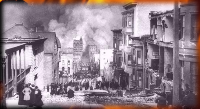
San Francisco Earthquake, 1906
