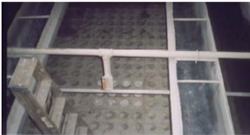
Figure 5-10. Underdrain System
