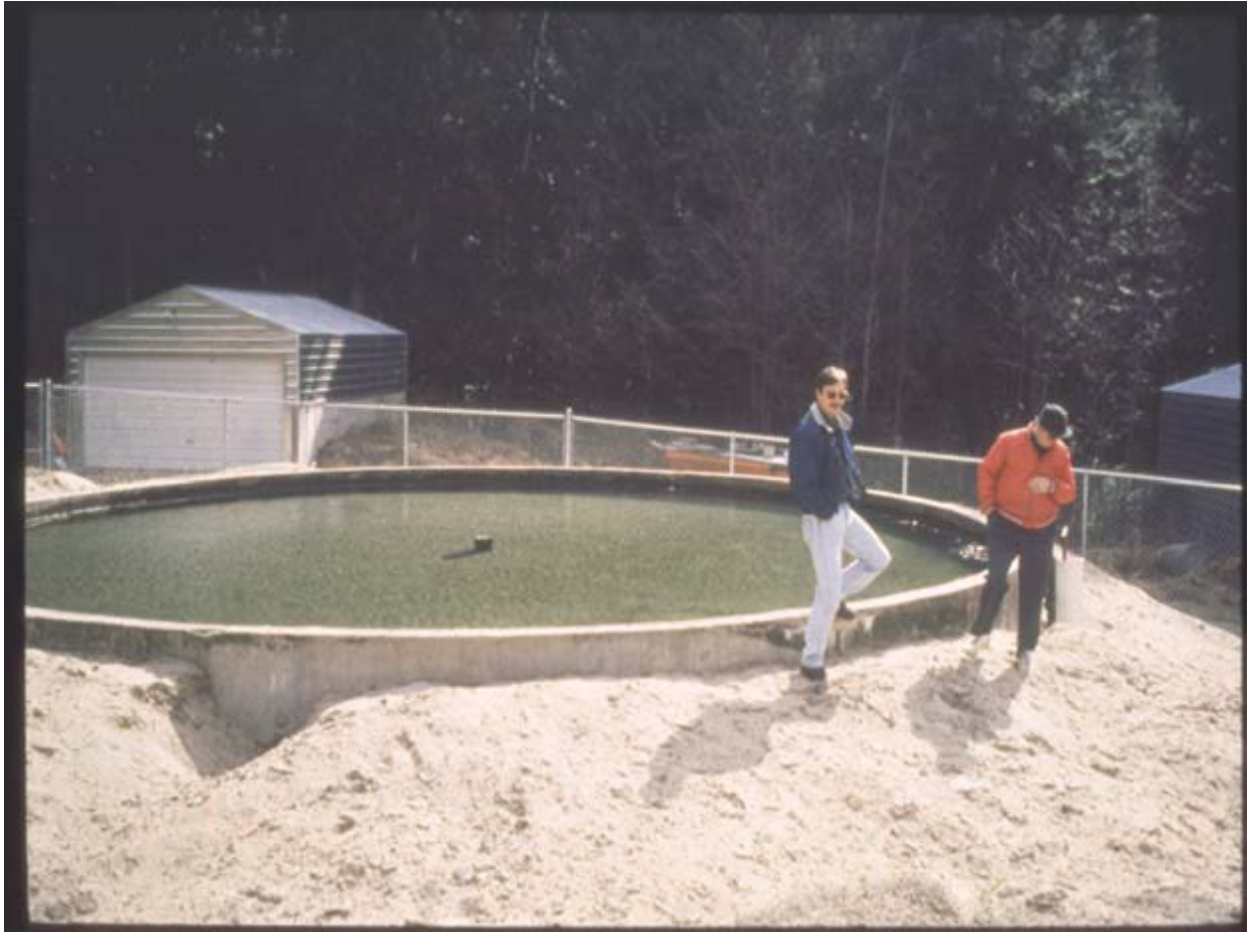
Figure 2-3. Slow Sand Filter in Idaho
