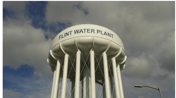
Flint Water Plant tower. (OIG photo)
