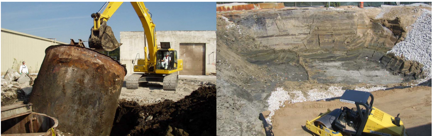
The 2004 to 2006 removal action.
