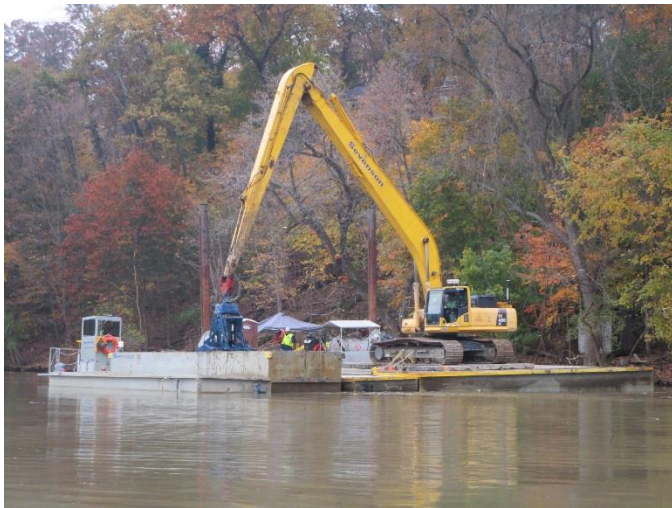
Sediment dredging underway near the "Island Area" of Pompton Lake.
