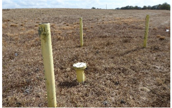
Monitoring well at the Site.
