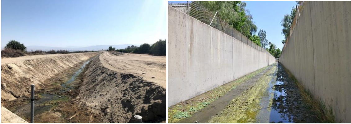
Figure 4. Examples of difficult conditions that may interfere with the observation or interpretation of indicators, such as hydrophytic plants. Note that even in the photo on the right, some vegetation is evident; field crews should determine if these plants are hydrophytes. In contrast, the photo on the left shows no vegetation due to the recent channel maintenance; in this case, returning to the site in a month or so may allow plants to recolonize the channel. Photo credits: Raphael Mazor.
