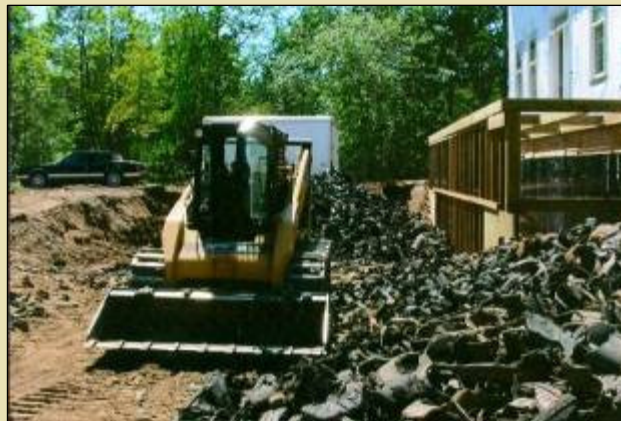
Residential foundation backfill
