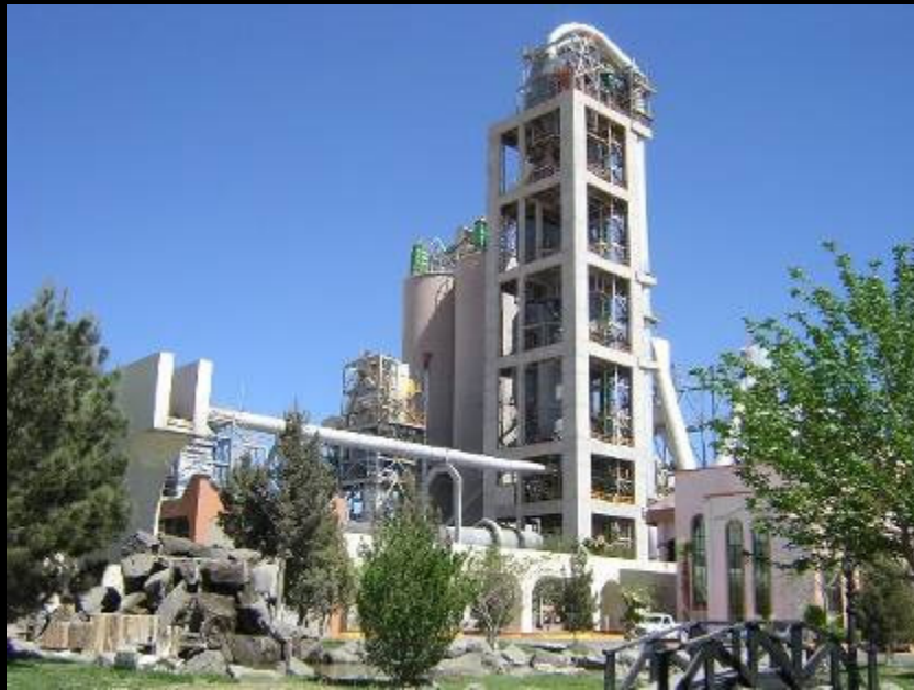
Cement Kiln in Juarez, Mexico.
