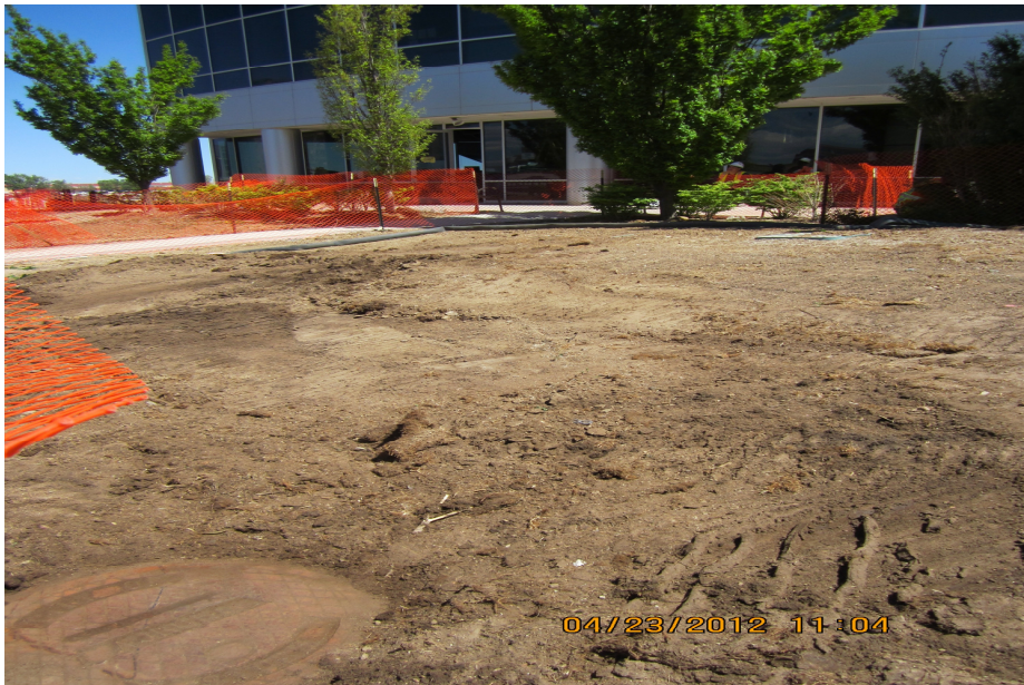
Outfall 001 (Latitude 39.740642 N and Longitude 104.830887 W) in relation to the Clinic Building South (CBS))
