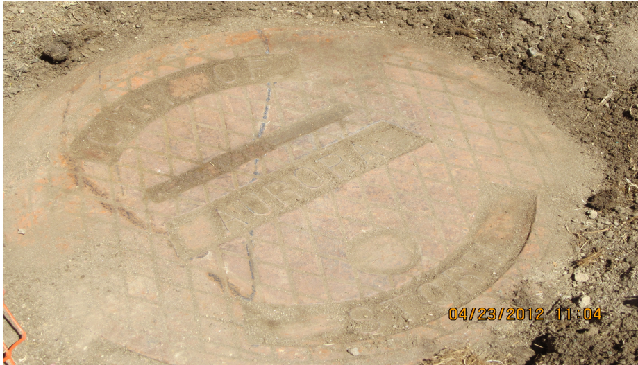
Outfall 001 (Latitude 39.740642 N and Longitude 104.830887 W)
