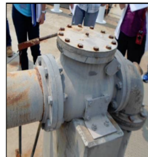
Kealakehe Pump Station Pump No. 2 Check Valve
