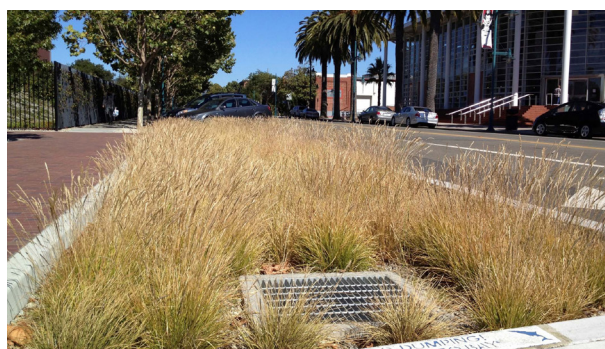
A “green street” uses practices such as porous pavement and bioretention to capture, infiltrate, and evapotranspire stormwater, preventing contaminated runoff from reaching local waterbodies.
