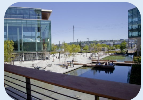
The Gates Foundation's 2-million-gallon capacity stormwater system in Seattle, Washington, collects and treats water from its central plaza and non-vegetative roof for flushing toilets, irrigation, and replenishing central plaza ponds.
