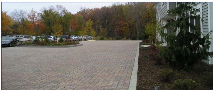
Image 10: Permeable paver parking lot at office building. (Photo courtesy of the final grantee report)
