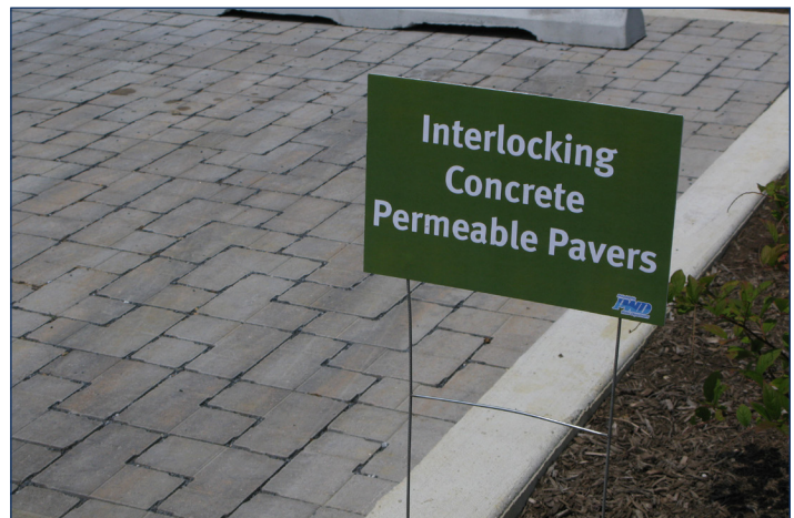
Image 28: Example of permeable pavements for increased groundwater recharge rather than surface water runoff in an urbanized area. (Photo courtesy of EPA)
