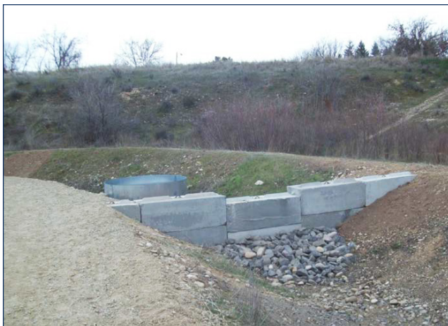
Image 6: Sediment basin dam at stormwater filter. (Photo courtesy of the final grantee report)
