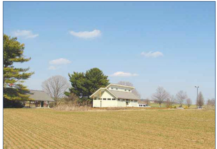
Image 22: Restroom facility, wetlands, and drip irrigation field. (Photo courtesy of the final grantee report)
