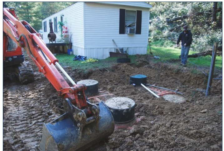
Image 27: Peat system installation. (Photo courtesy of Lincoln County Government)
