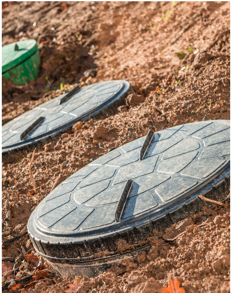
Image 1: Septic tank riser. (Photo courtesy of EPA)
