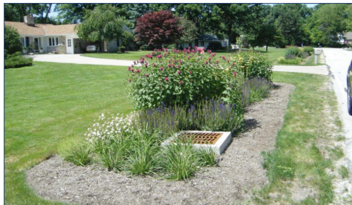
Image 12: Roadside bioswales along Fox Hollow Drive. (Photo courtesy of the final grantee report)
