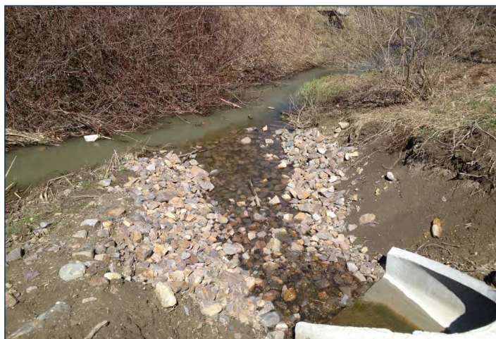
Image 35: Treated stormwater discharging from a retrofit detention pond. (Photo courtesy of the final grantee report)
