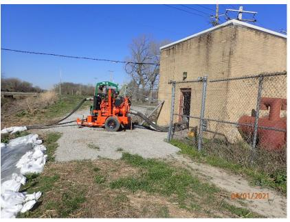
Description: Storm water pump station is being bypassed. Location: 68<sup>th</sup> and State Street.
