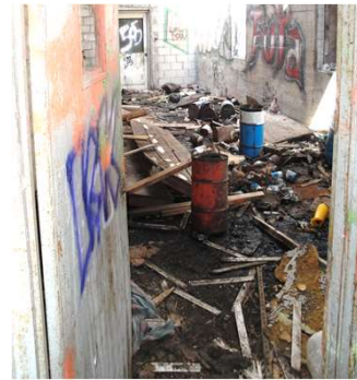
Assessment activities include site inspections to identify sources of contamination
