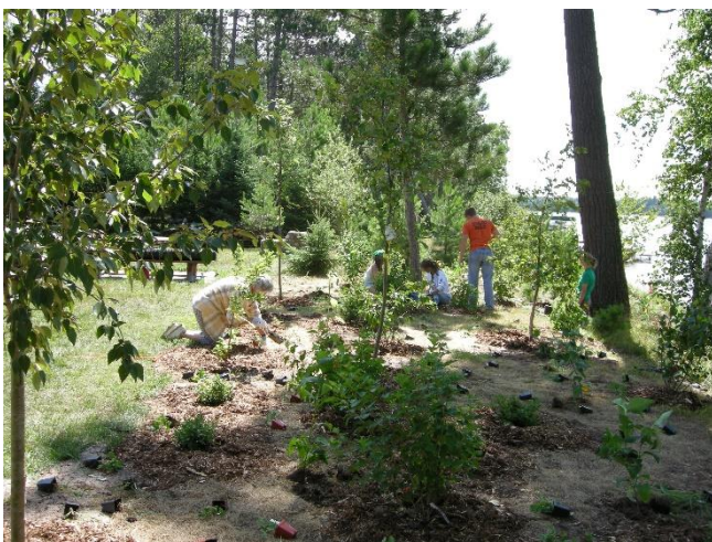
Shoreline buffer installation on a lake front property.
