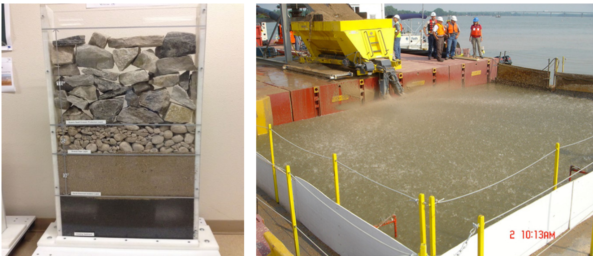
Figure 10. Photo of an engineered cap model and sand covering operations in the Lower Fox River (left credit Boldt Company, right credit JF Brennan)
