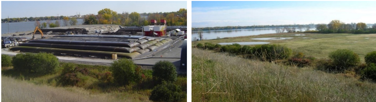
Figure 11. Left photo shows the OU1 geotube dewatering facility during active remediation and right photo shows the area post-restoration (credit Boldt Company).
