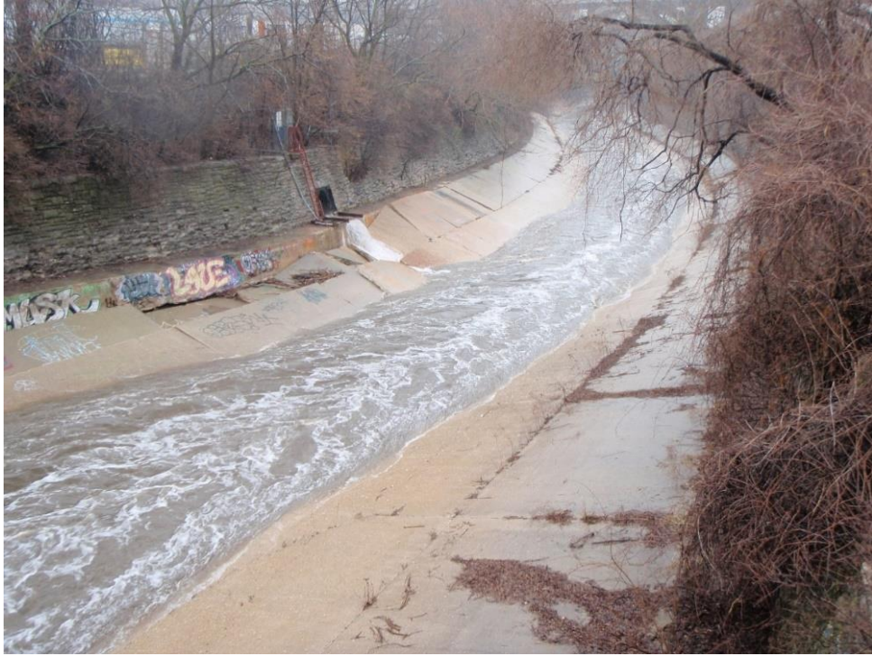
Figure 2. Concrete slabs along the Menomonee River before concrete removal (MMSD, 2013).
