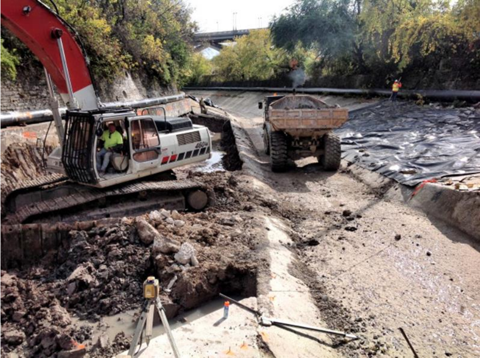
Figure 3. Removal of concrete slabs on the Menomonee River (MMSD, 2016).
