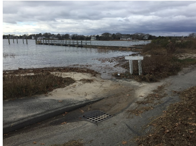
Bourne, MA: Circuit ave. flooding following storm. Credit: Timothy Lydon, Town of Bourne
