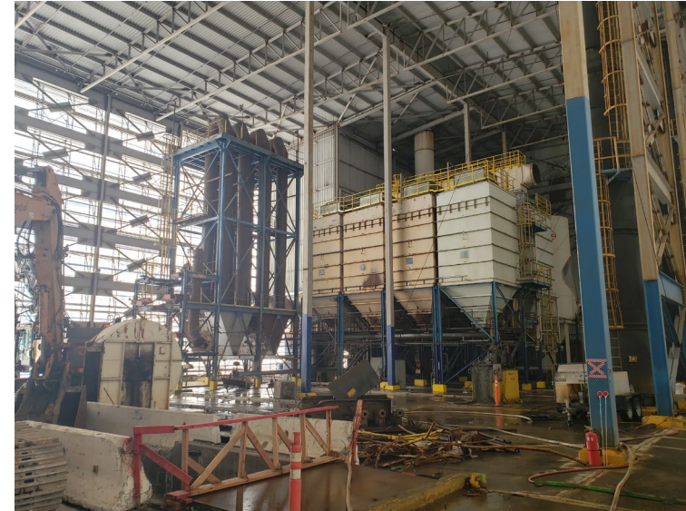
Segment 3 Baghouse Deconstruction
