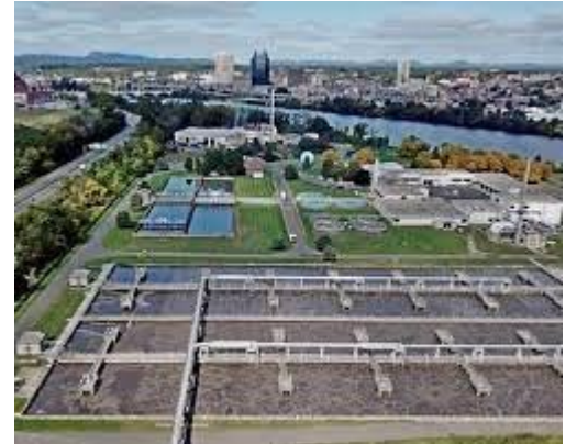
Photo courtesy of Springfield Water and Sewer Commission
