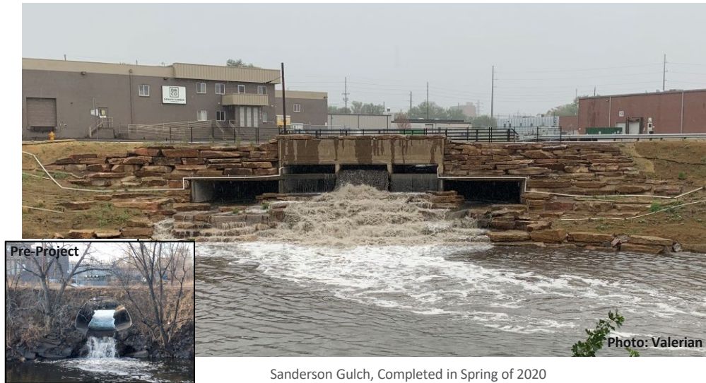
Sanderson Gulch, Completed in Spring of 2020
