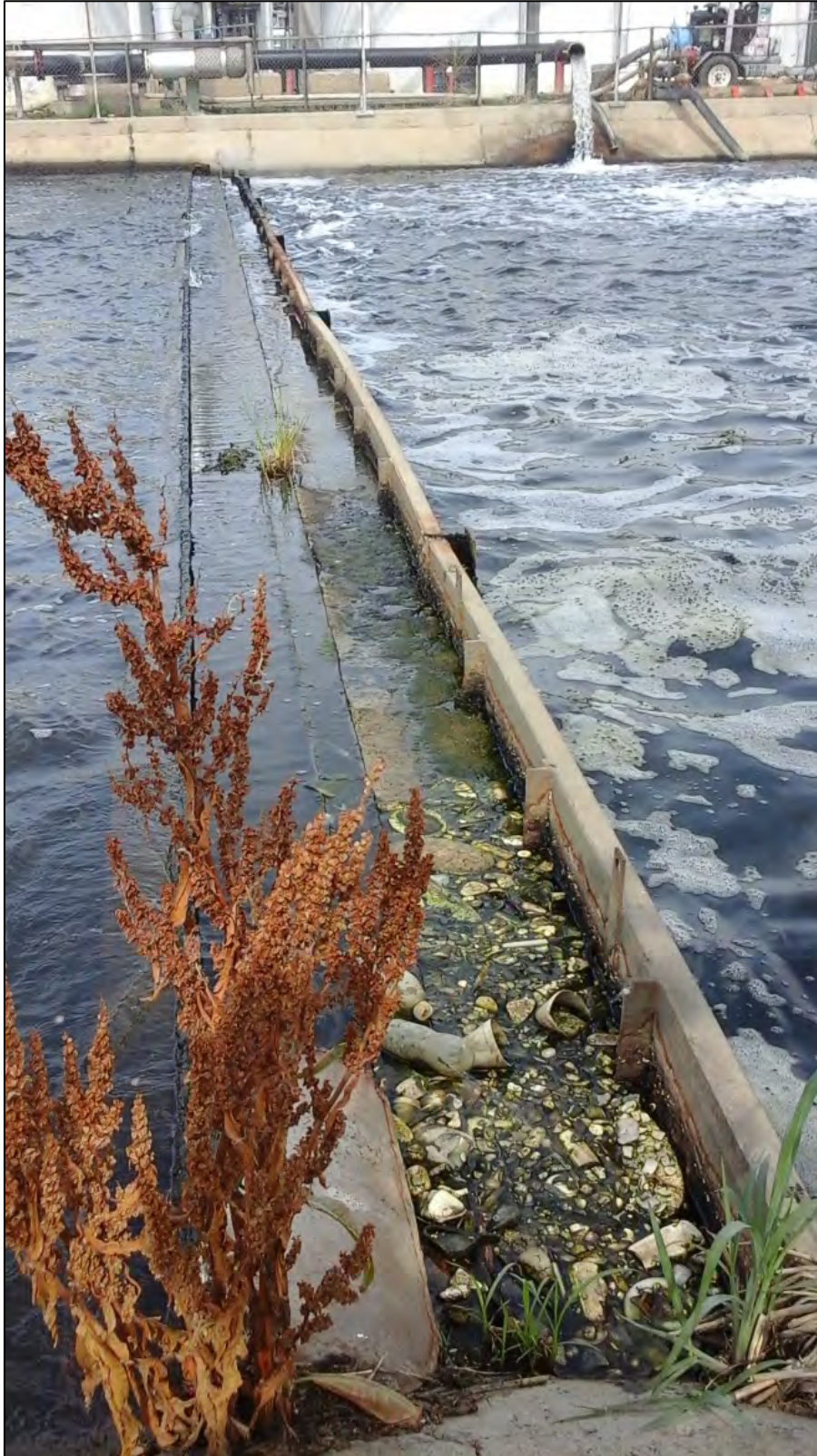
Photograph 12. View of accumulated solids and vegetative growth at the weir between Lagoon Nos. 2 and 3.
