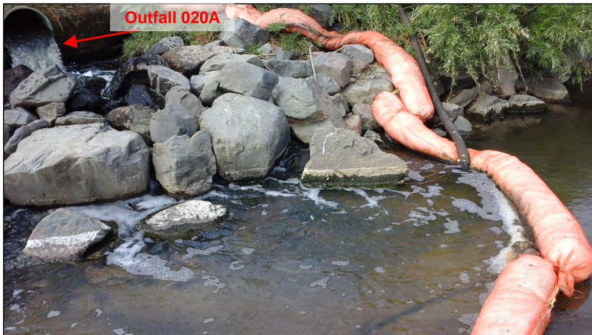
Photograph 2. Additional view of Outfall 020A to Sand Creek.
