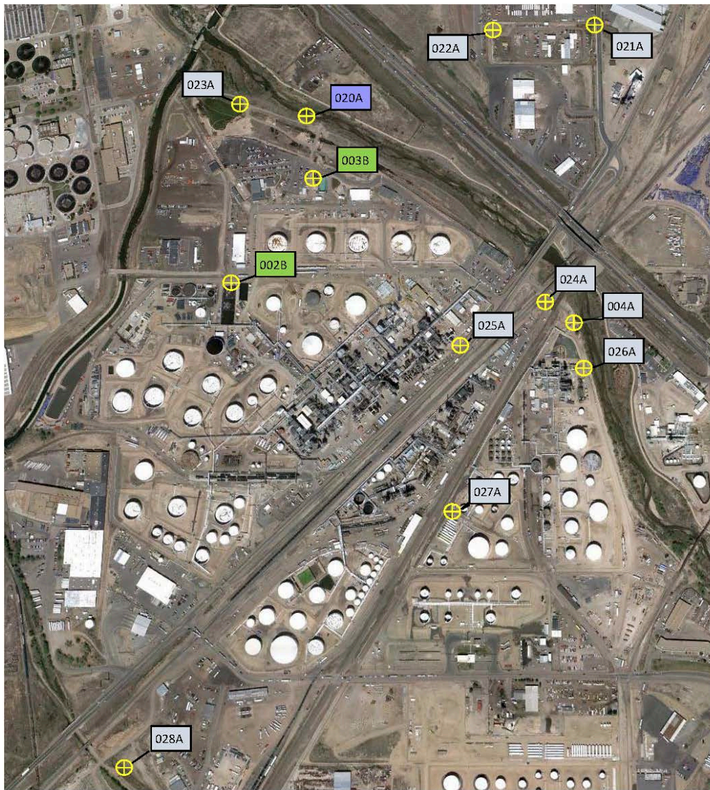
Figure 5—Wastewater and Stormwater Outfalls Suncor Energy Commerce City Refinery
