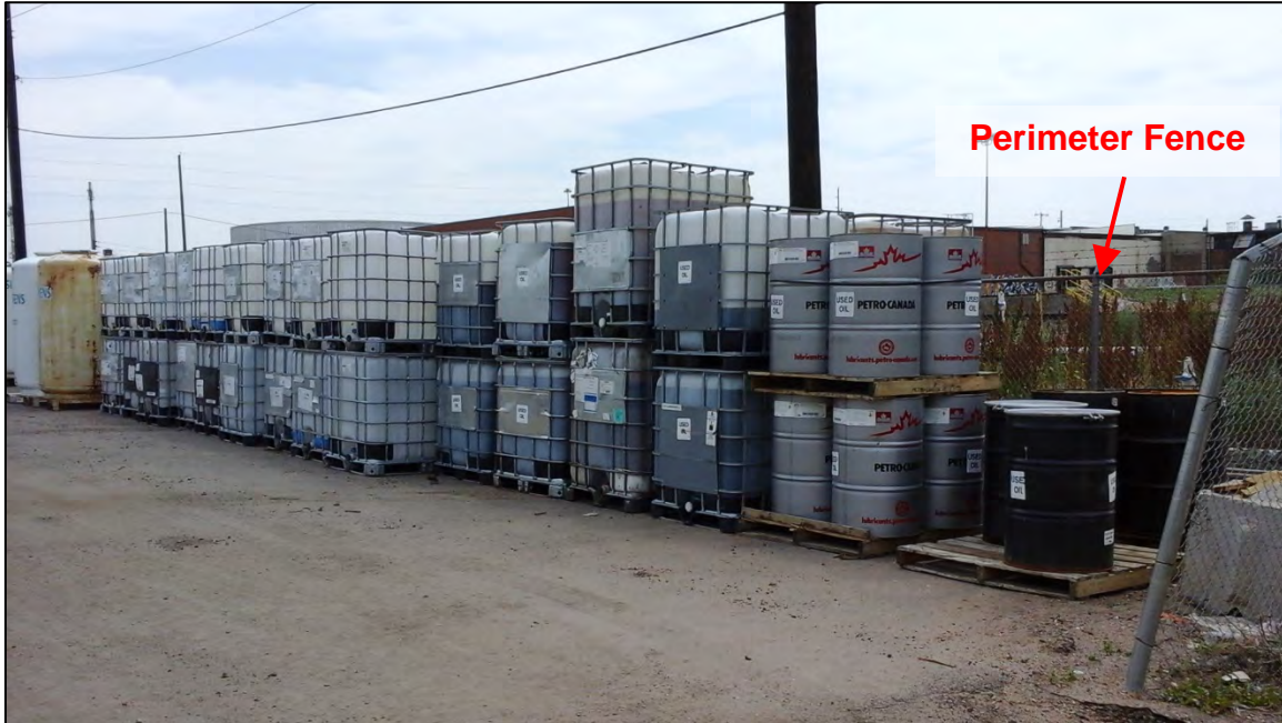
Photograph 25. View of waste chemical and used oil totes and drums storage area to the southeast of Webber's Pond. Secondary containment was not provided for these materials. Note the Facility's perimeter chain link fence.
