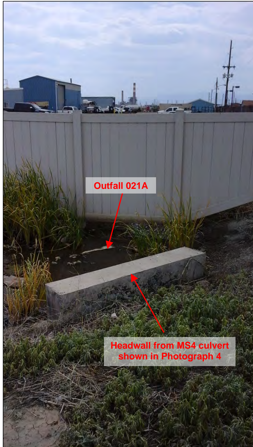
Photograph 3. View, facing west, from the Colorado Boulevard right-of-way, of Outfall 021A at the northeast corner of the Nelson Property. The stormwater detention basin on the northeast side of the property is located behind the white fence. Outfall 021A is noted as the location where accumulated stormwater is monitored and also where stormwater is commingled with stormwater runoff from the City of Commerce City’s MS4 from Colorado Boulevard.
