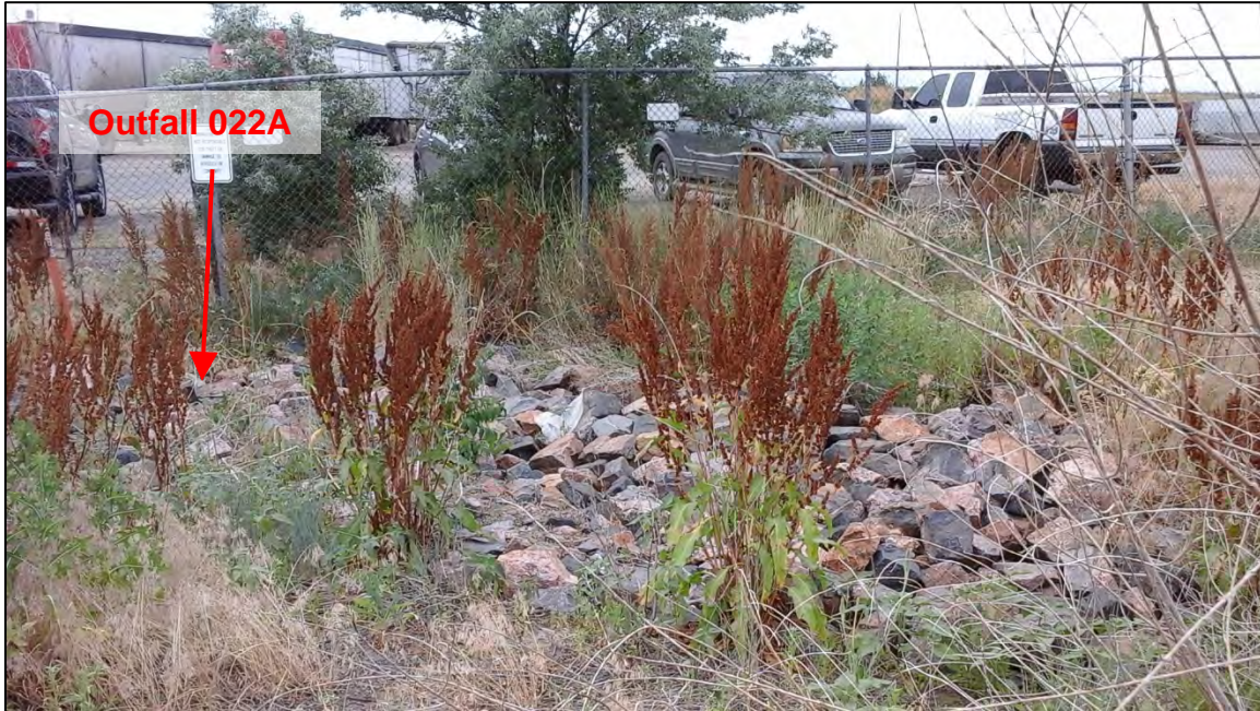
Photograph 5. View of Outfall 022A on the northwest side of the Nelson Property. This outfall drains into an adjacent offsite (behind chain link fence) parking lot and potentially to the City of Commerce City MS4.
