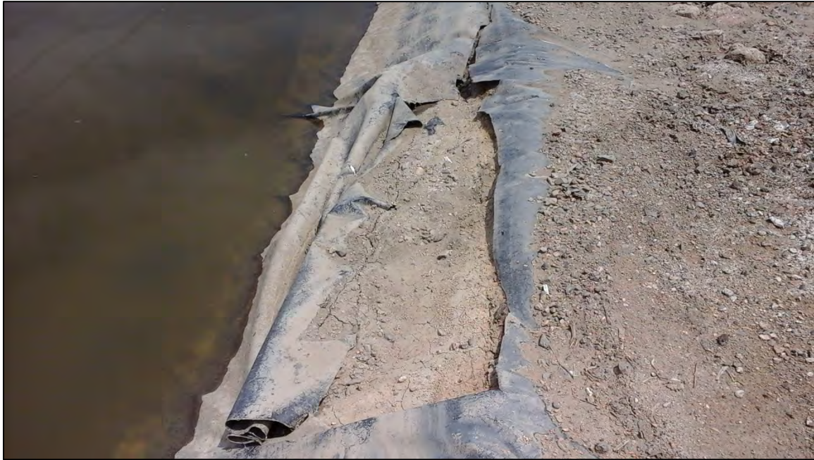
Photograph 36. Close-up view of the torn poly liner of Webber’s Pond shown in Photograph 33.
