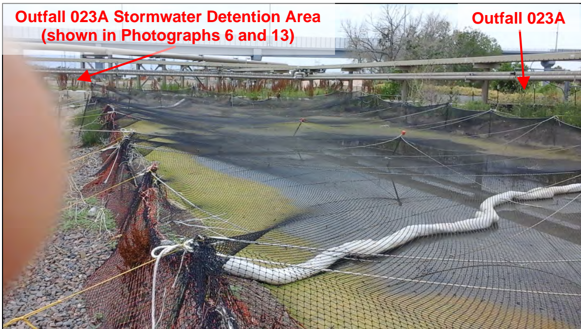
Photograph 12. View of the Sand Creek Swale Pond located between Plant 1 and Sand Creek where hydrocarbons during wet weather or times of elevated groundwater levels migrates to the ground surface. Note the black oil staining on the ground surface and netting to restrict wildlife access.
