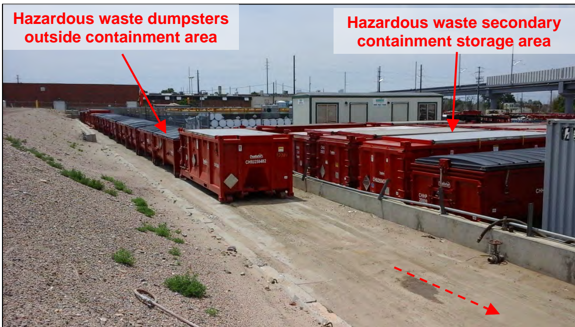
Photograph 37. View, facing southwest, of the hazardous waste storage area located in Plant 1, east of Webber’s Pond. Note six (6) red hazardous waste dumpsters were stored outside of this designated hazardous waste storage area and lacked secondary containment. Red dotted arrow indicates flow direction; refer to Photographs 38 and 39 for the observed flow pathway.
