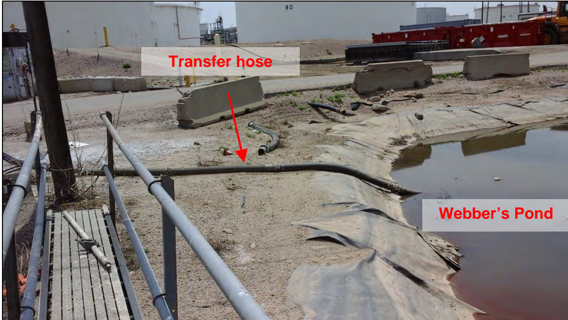
Photograph 21. View of transfer hose that connects Finger Lake and Webber's Pond.
