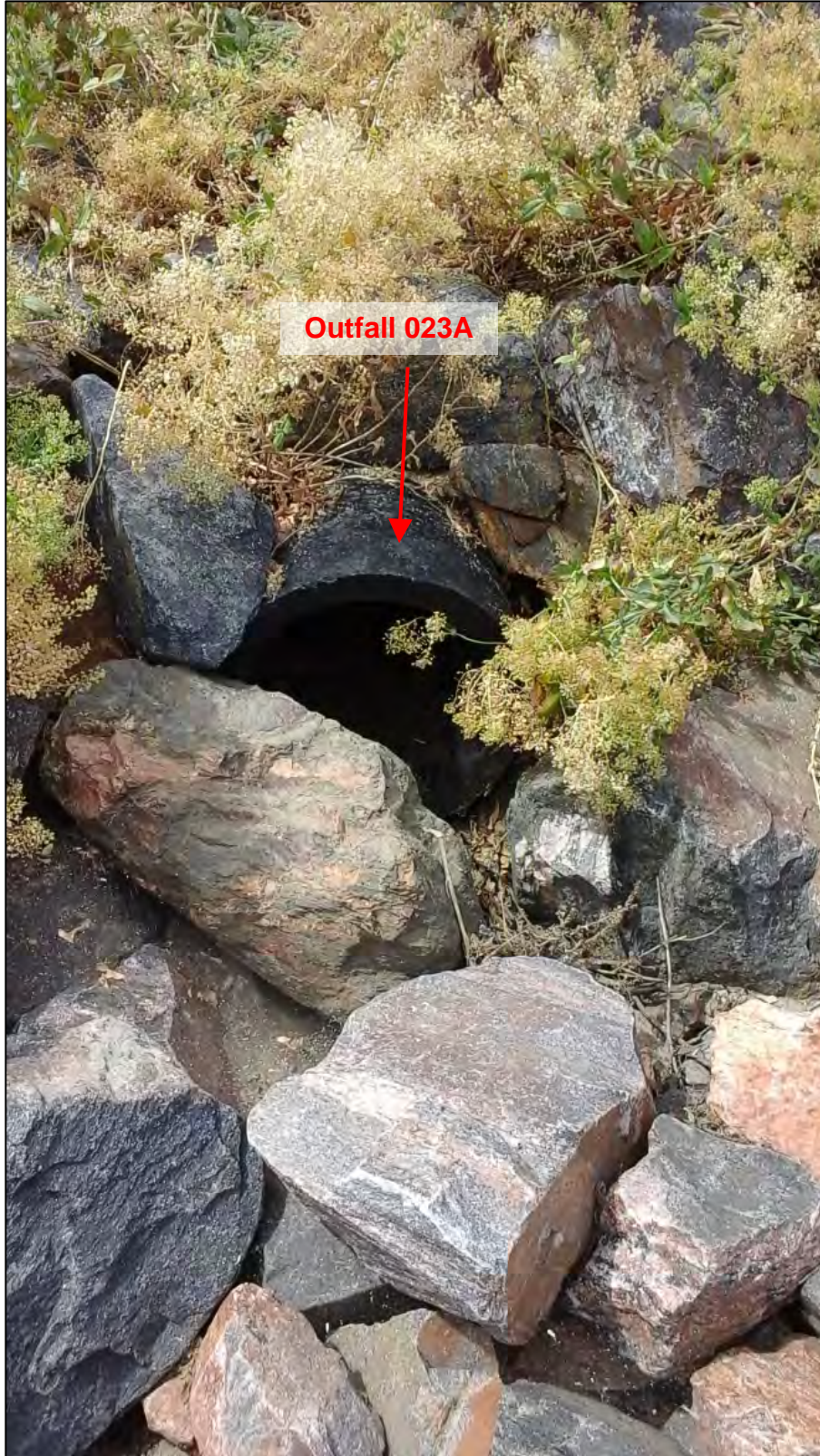
Photograph 7. Close-up view of Outfall 023A from stormwater detention area, shown in Photograph 6, which discharges into Sand Creek.
