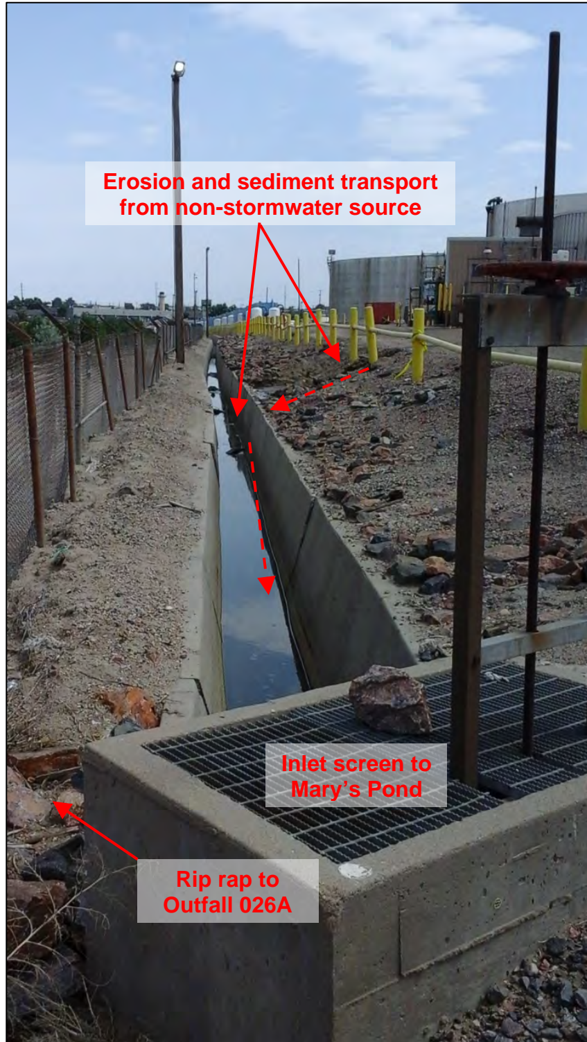
Photograph 31. View, facing south, of evidence of erosion occurring upgradient of the Plant 3 east perimeter concrete channel that leads to Mary's Pond (Outfall 004A) or to Outfall 026A during high flow events. Red dotted arrow indicates flow direction. According to Facility representatives this continual flow was from non-contact cooling water in Plant 3 into this channel. Note the slope above the channel was eroded due to the continual flow.
