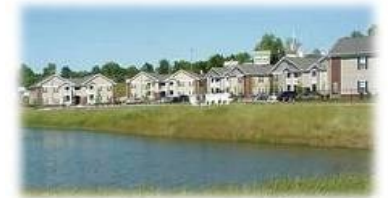
After: Union Mill – Union, South Carolina
