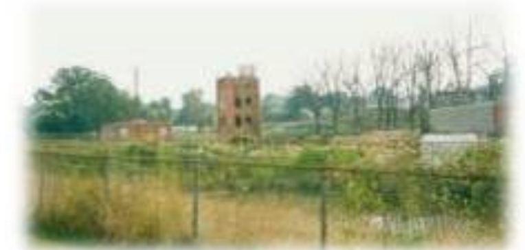
Before: Union Mill – Union, South Carolina
